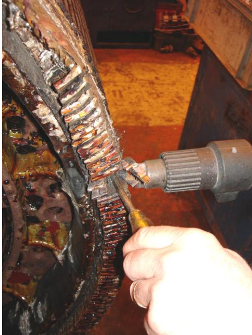
Heat-gun softens up the windings to ease prising them out. Photo by Mike Jacob.
