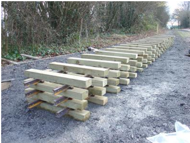
Track panel production 20 th February.
