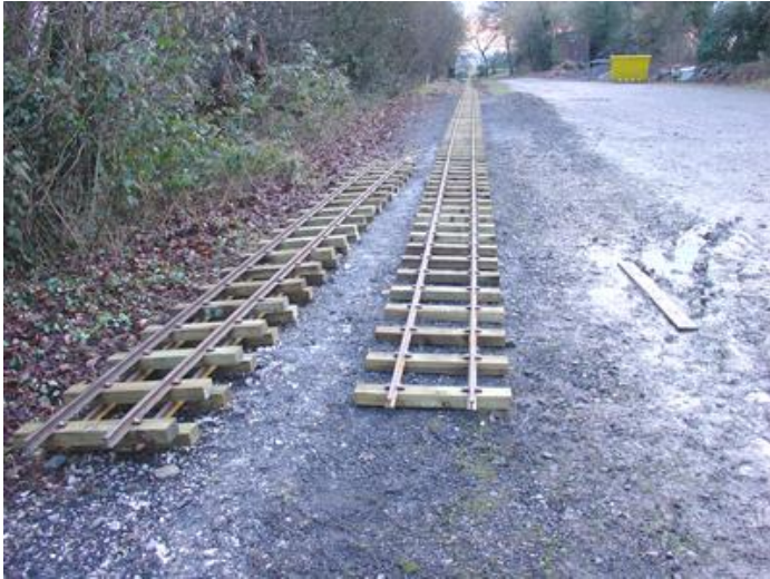
Track panels being placed in position 28 th February.
