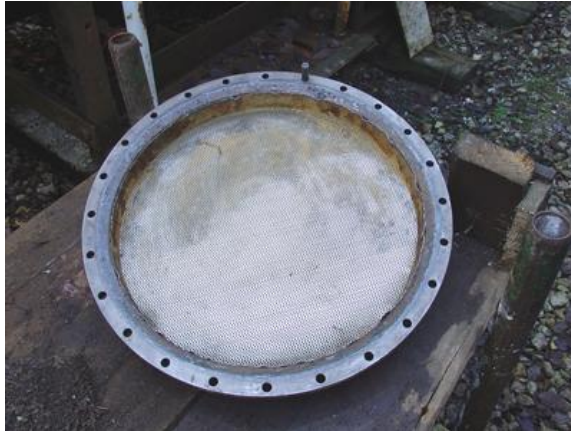
Intercooler end cover undergoing cleaning.
